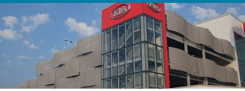
Curved structures used to produce a unique and long lasting feature decorative mesh facade at the new flagship Kia Motor dealership in London.
