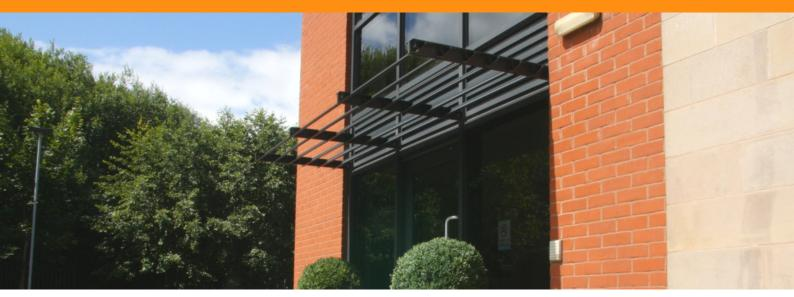
Large profile commercial solid blade manufactured from extruded aluminium. The pitch varies depending upon the projection and orientation of the installation. Overall a strong blade which can span up to 1.8 metres between supports.
