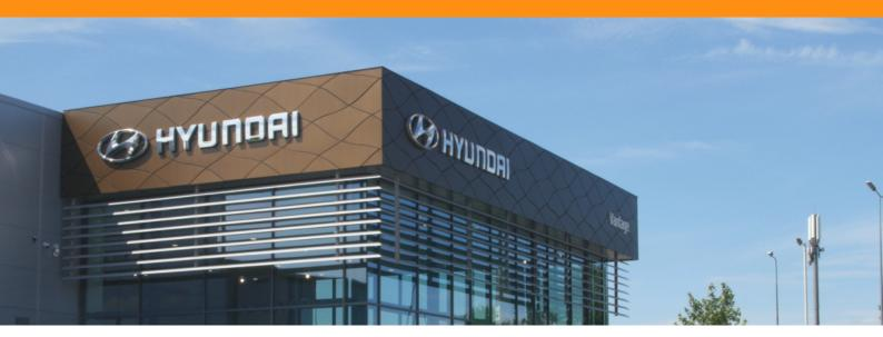
WPL's Aerofoil range comes together to form a fixed aluminium solar shading system.
