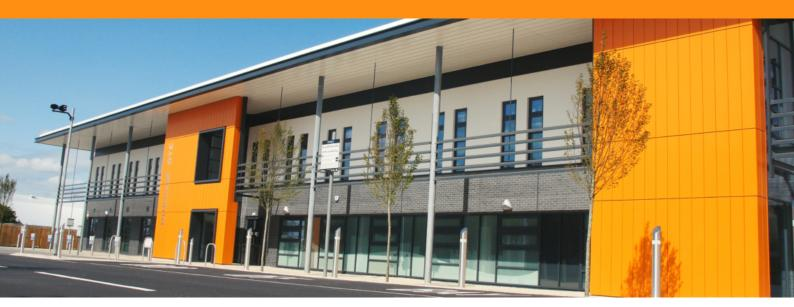
At Durham's NHS Diagnostics and Treatment Centre the designers diagnosed a potential overheating issue caused by direct sunlight through the windows. WPL's antidote was the inclusion of AF200 aerofoil system over the glazed areas.
