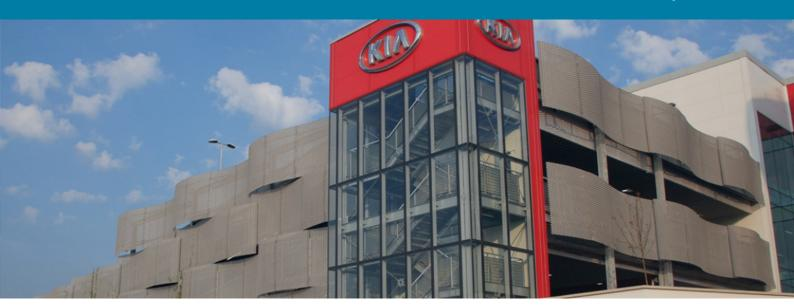
Curved structures used to produce a unique and long lasting feature decorative mesh facade at the new flagship Kia Motor dealership in London.
