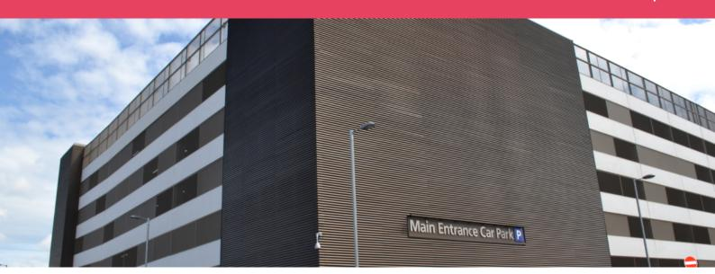
A small profile manufactured as a continuous or panel form for rain defence with good ventilation. The strucuture of the blade minimises air pressure losses which drive essential ventilation, yet still protect the area from unwanted water entry.
