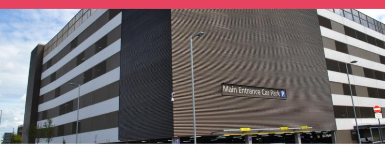
The new MSCP required a feature louvre system as part of the overall design package at the Blackpool Victoria Hospital.
