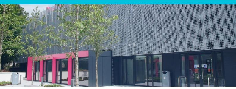
At the Arts University Bournemouth WPL designed and installed a perforated rainscreen cladding with perforations of differing positions and diameter. The final effect produces a unique facade which was repeated across different campus buildings.
