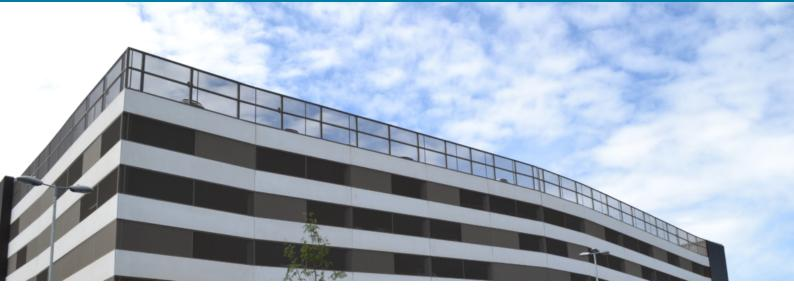
At Blackpool Victoria Hospital's MSCP an expanded mesh was custom designed, manufactured and installed to deliver on an aesthetically pleasing feature within the technical parameters of the national car park guidelines for ventilation and light entry.
