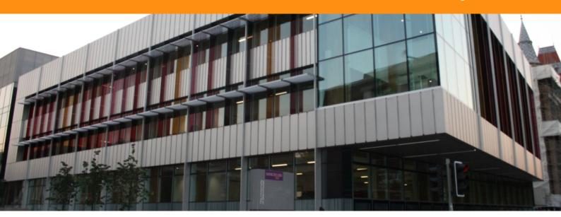
To design, supply and install horizontal projected Solar Shading fixed back to feature glass laminated fins on the University of Manchester's Learning Commons Building.
