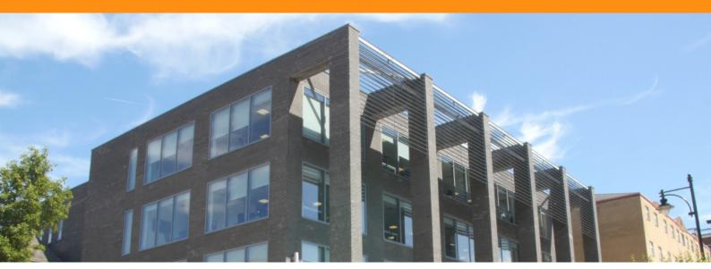
First Choice Homes built a new HQ in Oldham town centre which incorporates an array of WPL products. Solar Shading at high level using WPL's aerofoil range with a feature handrail and balustrade to the pedestrianised balcony along with extensive louvred walls and doors at low level.
