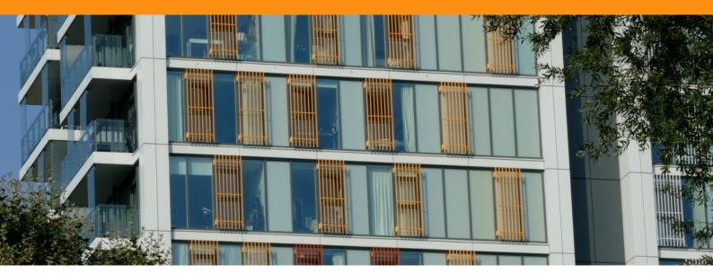
W P L supplied vertical extruded frames to the external facades which assist in making the lived-in environment more private for the occupants of this luxury real estate in London. The feature was enhanced by mixing the colours with a gradual change from deep red to yellow.
