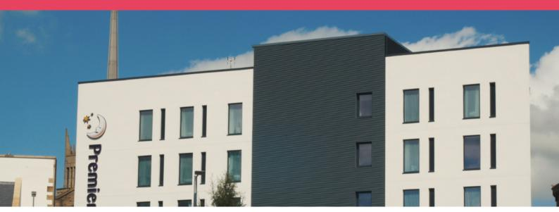
At the 60-bed Premier Inn and the new six storey offices at Cathedral Quarter in Blackburn louvre panels and doors were incorporated to add an extremely striking feature on one building from ground level right up to the rooftop and functional louvres and doors at ground level on the other building.
