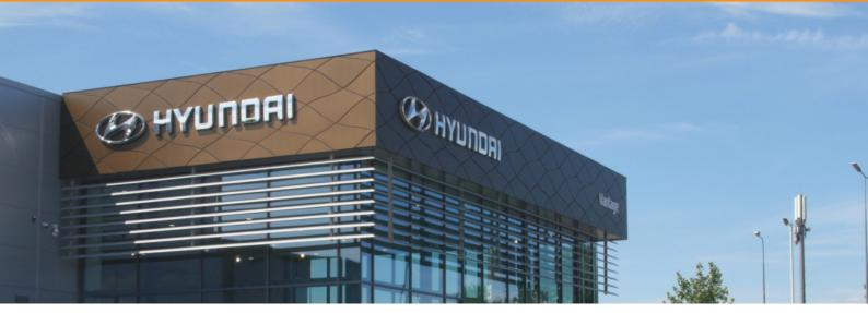
WPL's Aerofoil range comes together to form a fixed aluminium solar shading system.
