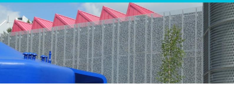
Rainscreen cladding panels with perforations of differing positions and diameter.
